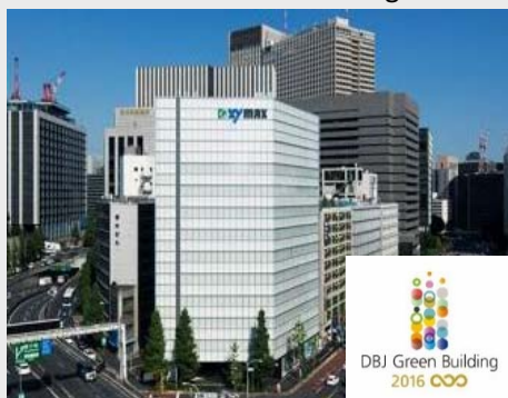
XYMAX Akasaka 111 Building*
